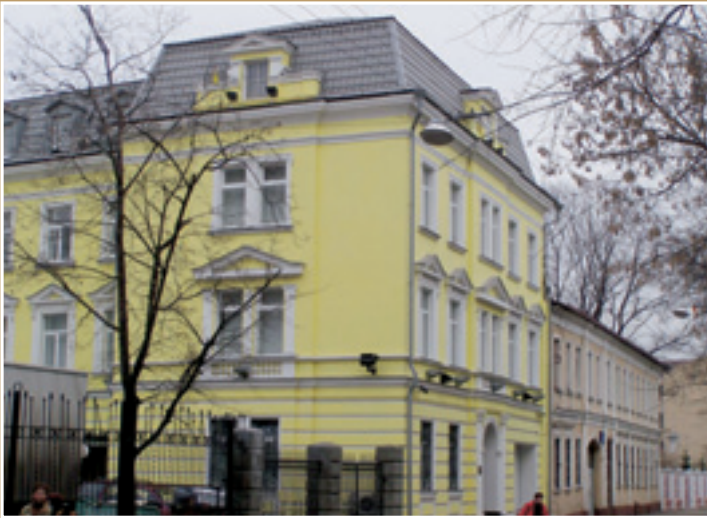
The new client centre – Central Additional Office
